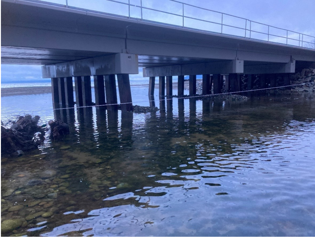
Figure 8. Tidal inundation upstream of the former railroad culvert, January 25, 2023. Predicted tidal elevation was 12.54 ft MLLW, though actual tidal elevation was estimated to be 11.63 ft MLLW based on gauge data. The NAVD elevation recorded on the staff gauge was 9.6 feet.
