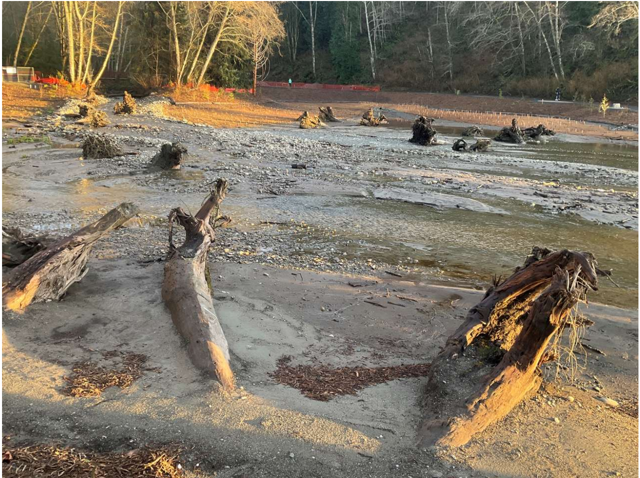
Figure 3. Lund's Gulch Creek excavated embayment area looking upstream toward the creek mouth (with trees), the alluvial fan with riffle habitat in creek segment 2, with large woody material placed in the embayment area. Woody material is inundated at higher tidal elevation.
