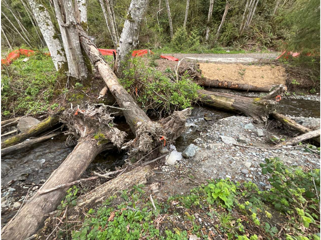
Figure 7. Large Woody material (flagged) with rootwads placed in Lund's Gulch Creek in creek segment 3.
